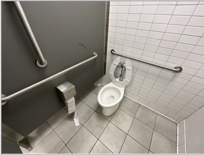
TOILET STALL OVERVIEW
